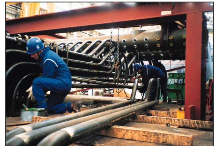
Fabrication of Feeder/Header Assembly
