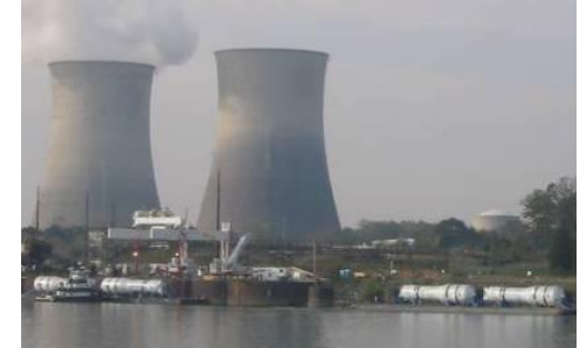
Watts Bar #1 Steam Generator
